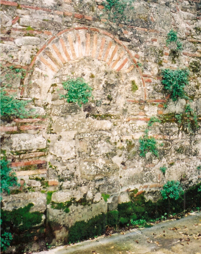
Fig. 62. Ag. Georgios, Ag. Georgios. Sections of masonry in the: A) S façade, B) N façade.
